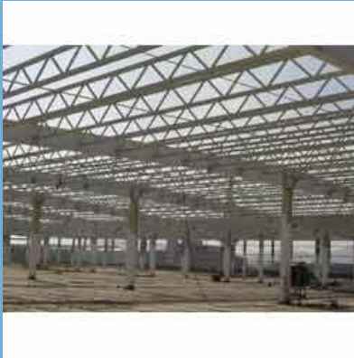
Roof Truss Fabrication
